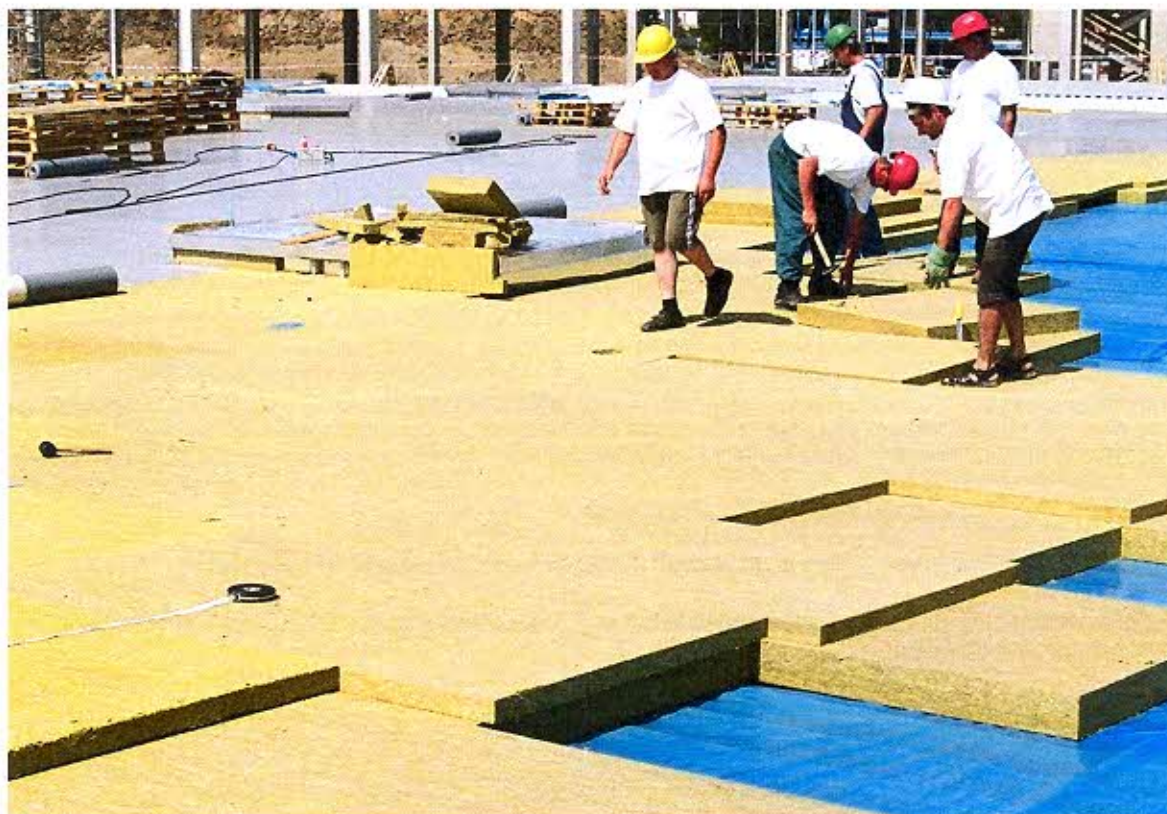
Isover S as a top layer on flat roof mineral composition.
